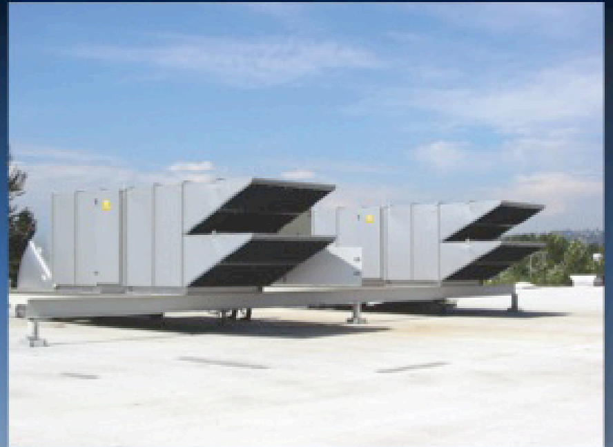
Roof Mounted Units With Evaporative Coolers
