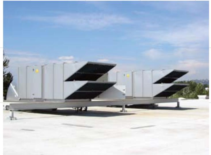
Air make-up units with temperature and humidity control for critical applications
